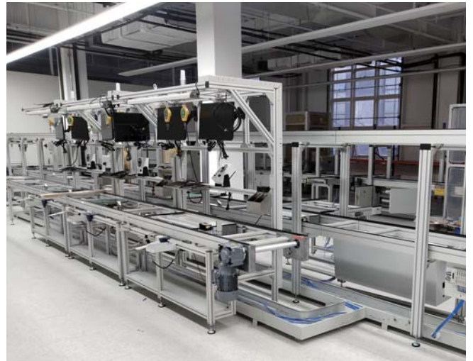
Pallet conveying control system 托盘输送控制系统
